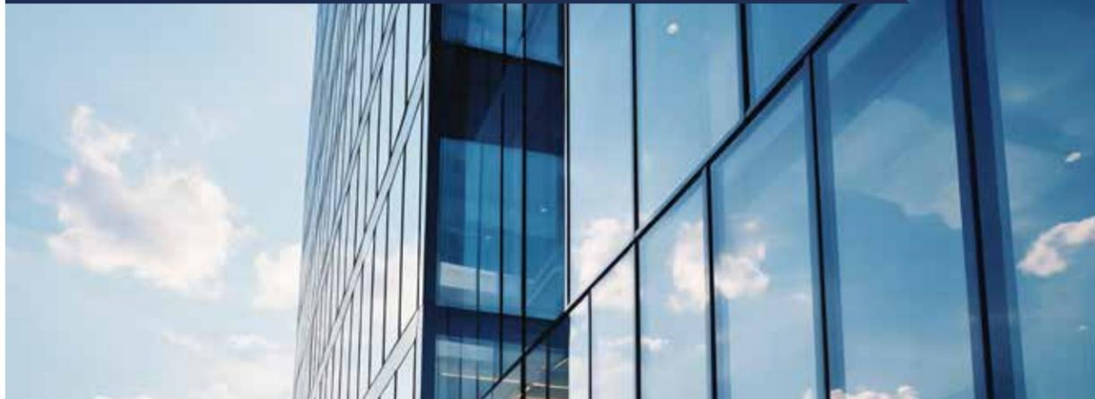
Insulated glass is a glass product in which two or more pieces of glass are evenly separated by effective support, and the periphery is bonded and sealed to form a dry gas space between the glass layers.
